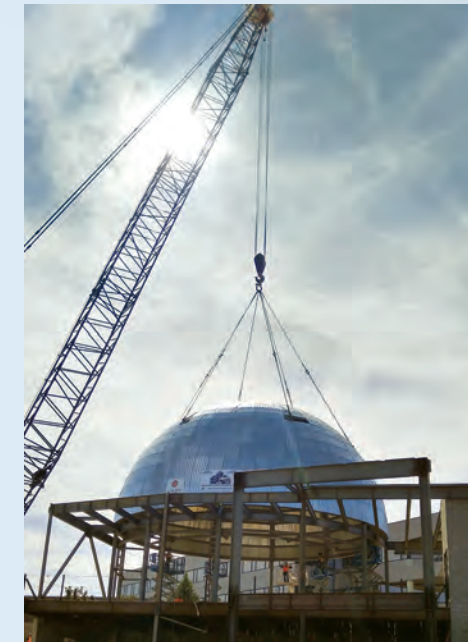
Raise the Roof: It took three hours to install the planetarium’s 220-piece, 127,000-pound steel dome.
